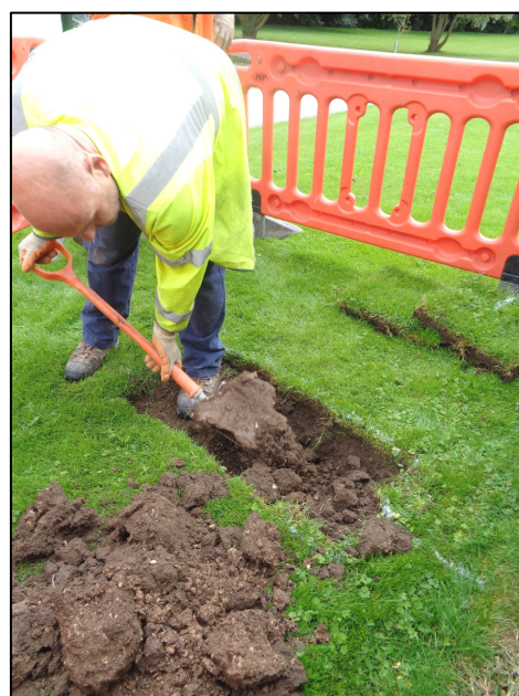
Plate 2: Hand excavation of Test Pit 3.
