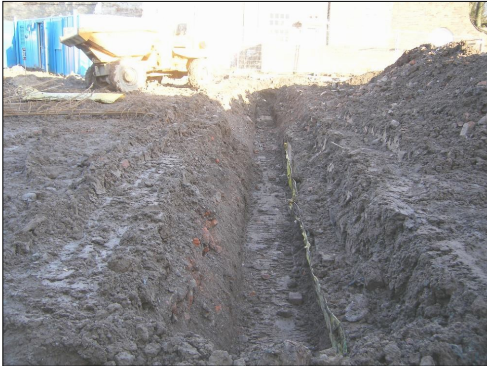
Plate 5: View of made ground in drainage trench looking west
