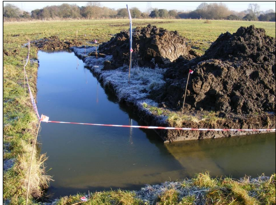
Right: Trenches flooded soon after excavation due to high ground water. Trench 9.
