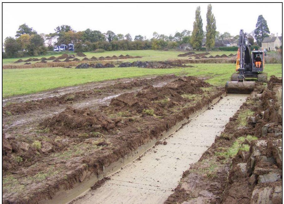
Above: Site during trench excavation; Trench 8 in foreground.
