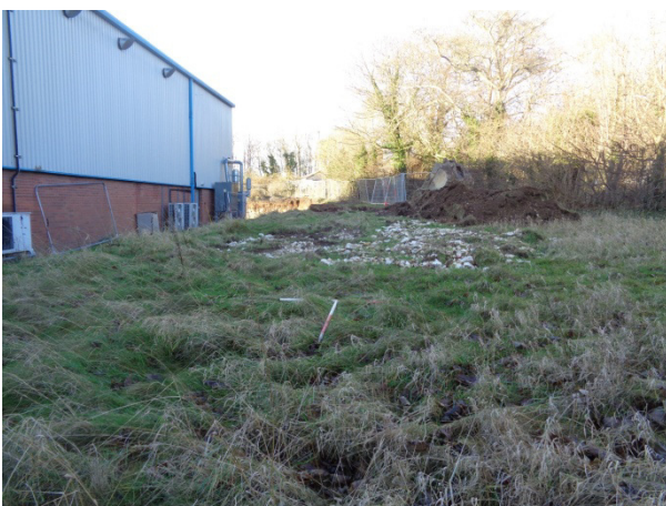
Plate 7: Pre-excitation shot of area to the north of existing warehouse (looking W).
