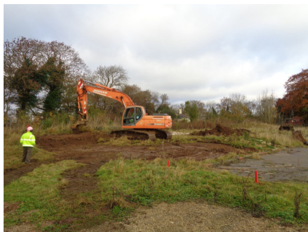
Plate 2: Working shot of western side of development area (looking NW).
