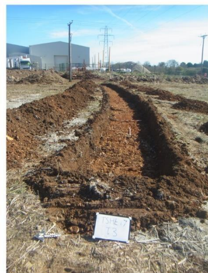
Plate 5: Trench 3 (looking E)
