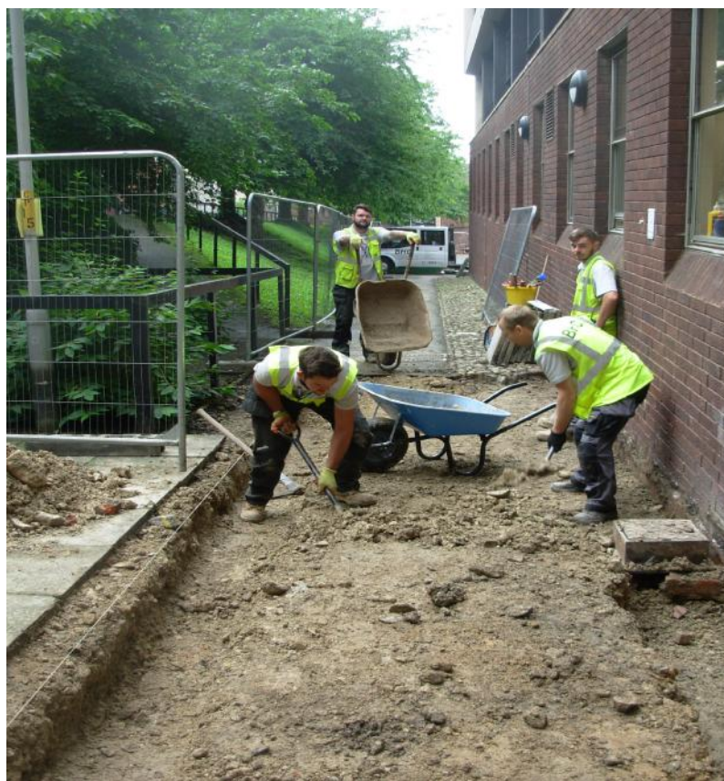
Plate 3: Working shot; lowering ramp area facing south.
