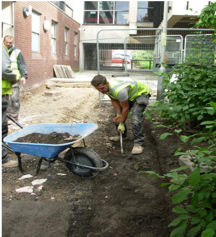
Plate 6: Excavation of bank topsoil, looking north
