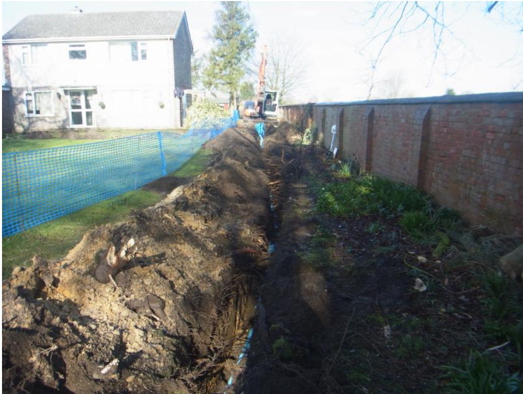
Plate 1: Excavation of service trenches
