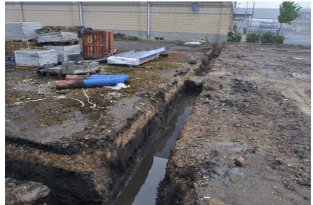
Plate 2: Foundation trench (looking NE).
