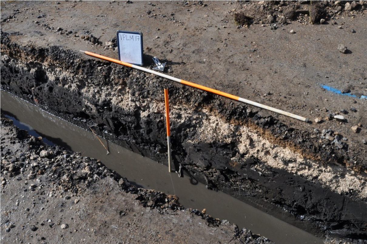
Plate 5: Representative section of foundation trench (looking S). See Fig. 3.
