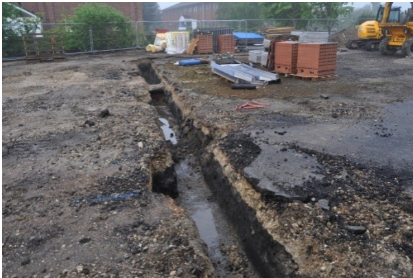
Plate 1: Foundation trench (looking SW).
