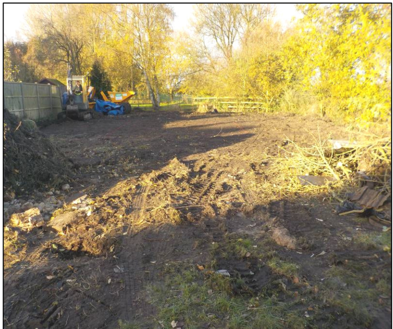
Plate 1: General view of site looking west
