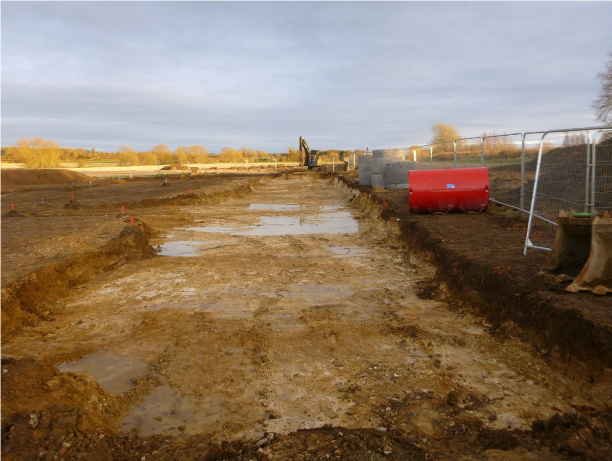
Plate 5: Further working shot of site strip (looking E).
