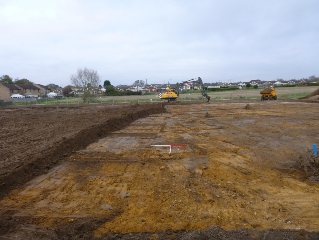
Plate 4: Working shot of site strip (looking N).
