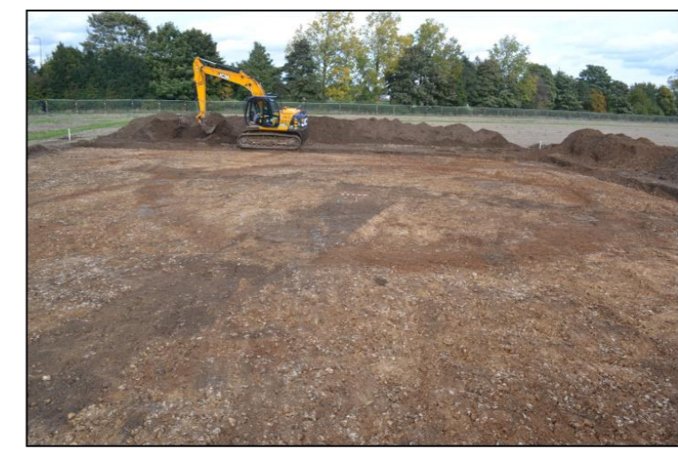
Plate 1: Overview of Excavation Area after initial site strip
