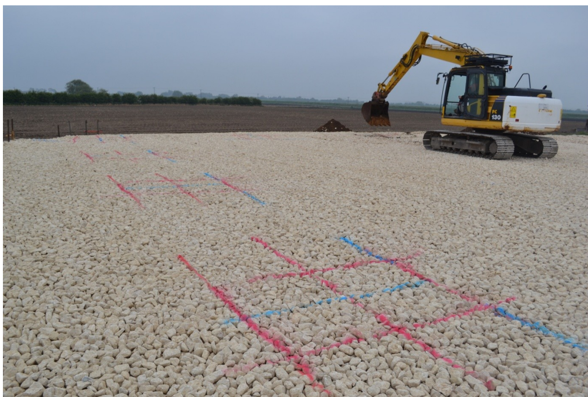
Plate 4: Working shot during second day of monitoring (looking SSW).
