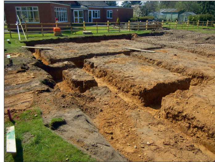
Looking west across the excavated footings of the new dwelling
