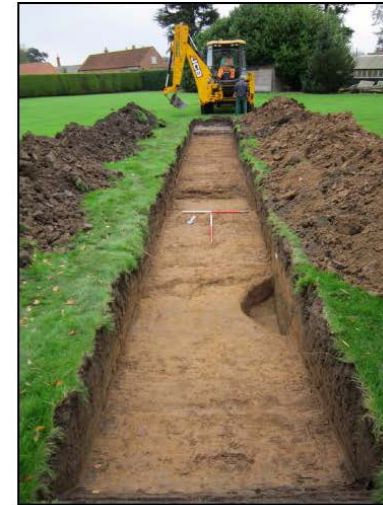
Plate. 1: Looking south along the excavated trench
