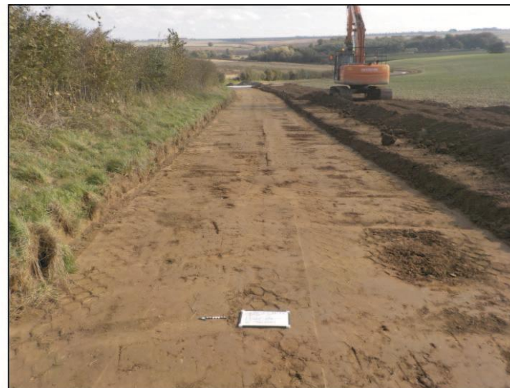
Plate. 2: Looking east c. 550m along the new access track
