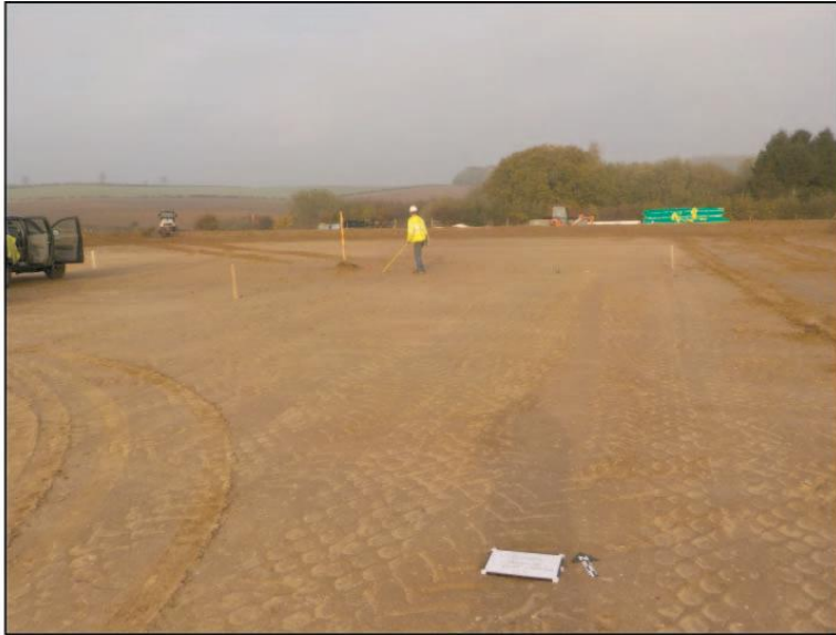
Plate. 5: Looking north at area of well site after initial site strip
