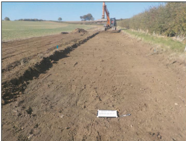
Plate. 1: Looking west along the new access track during machine strip
