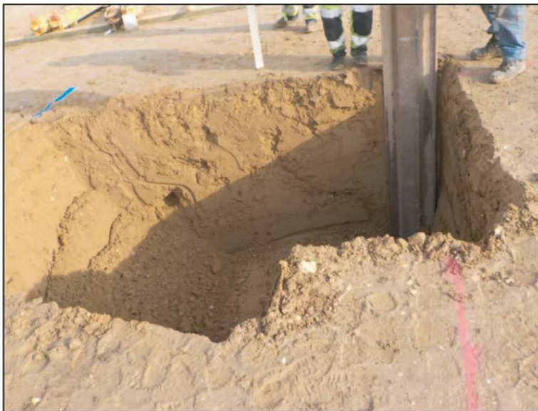
Plate. 7: Looking north at Well Site Cellar excavation
