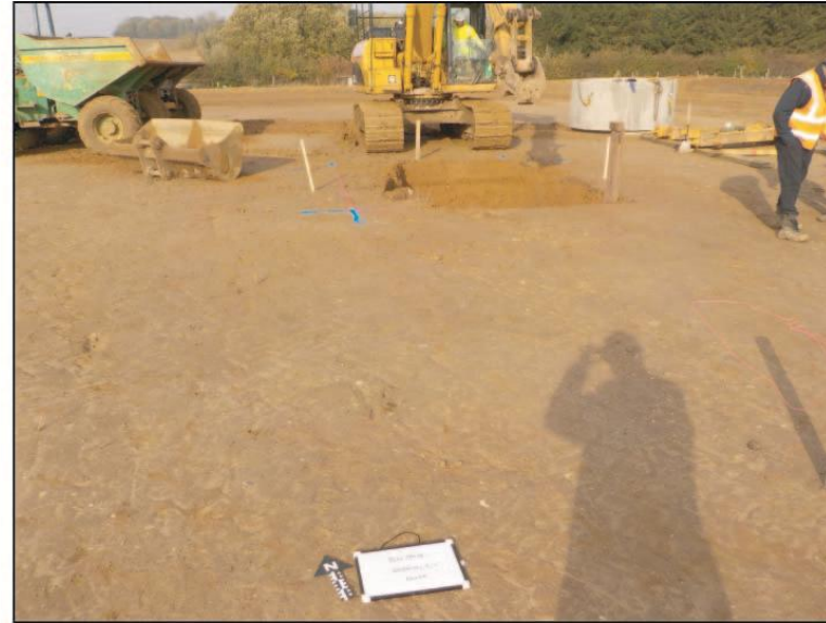
Plate.6: Looking north during the excavation of the Well Site Cellar
