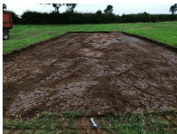
Plate 2: Complete topsoil strip (looking SSW)
