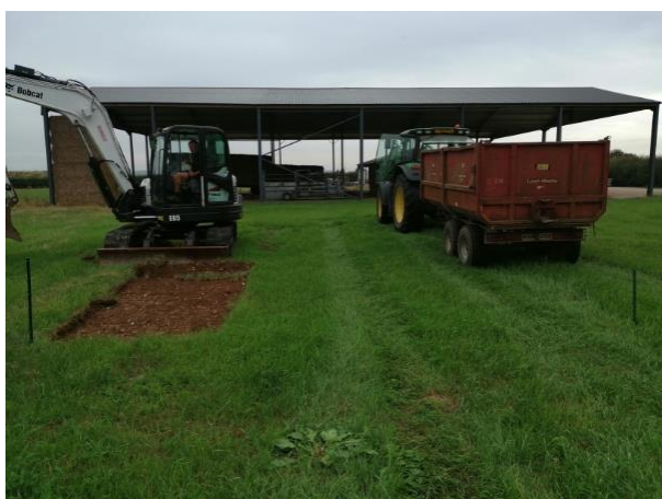
Plate 1: Working shot of topsoil strip (looking NNE)
