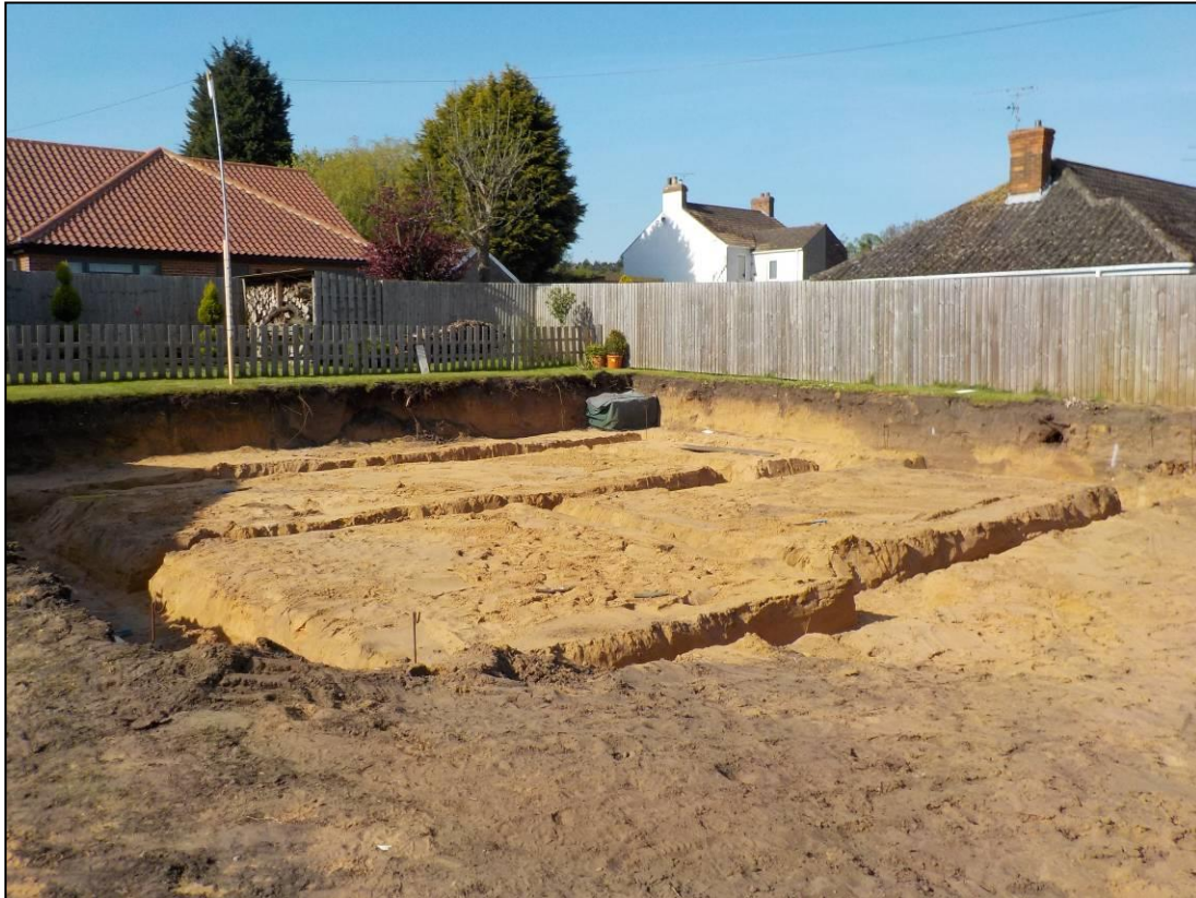
Above: New bungalow footings excavated into natural geology
