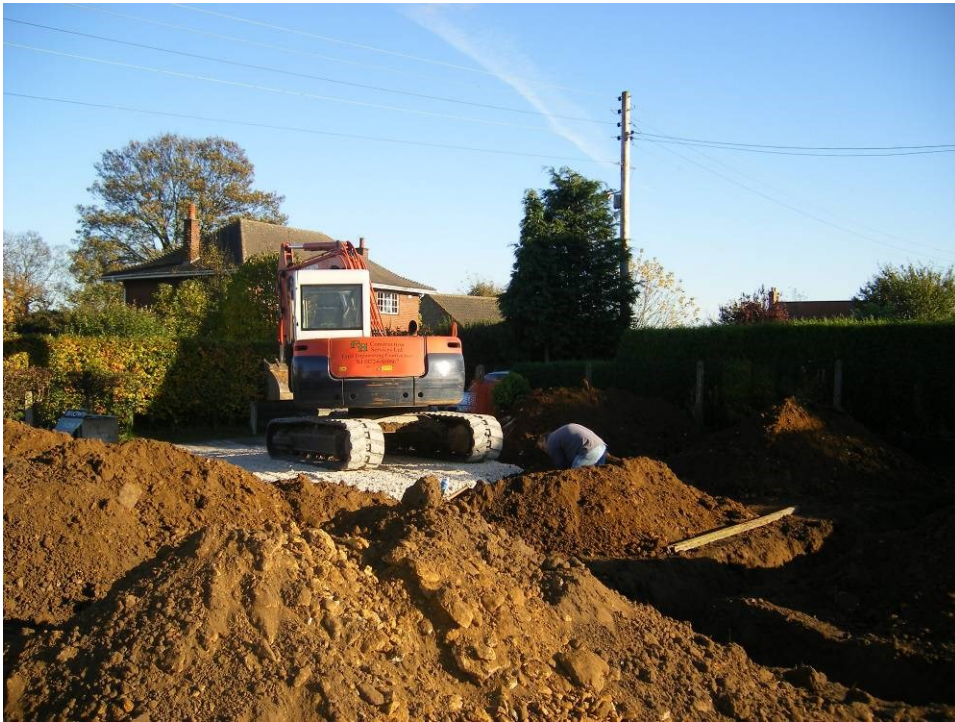
Plate 1: General view of site looking south east
