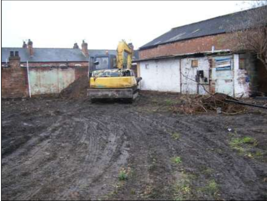
Plate 1: General view of site looking west
