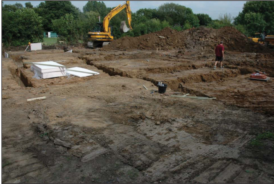
Plate 1: General site view looking north east
