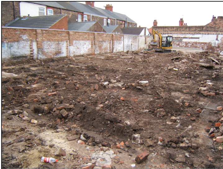
Plate 1: General view of site looking south.
