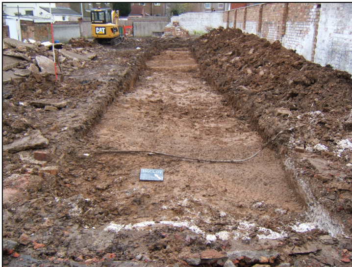
Plate 2: View showing excavated trench with ditch [003] in the foreground, looking north-east.
