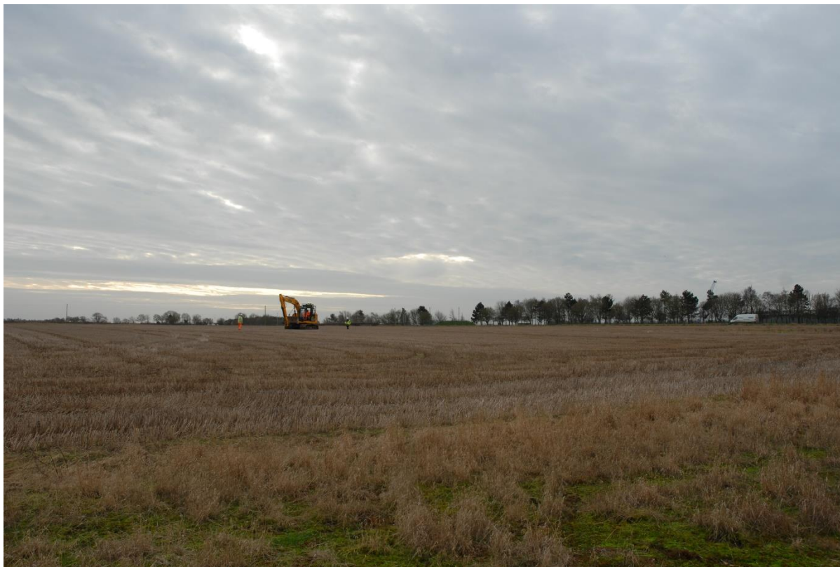
Plate 1: Site prior to excavation (looking SW)
