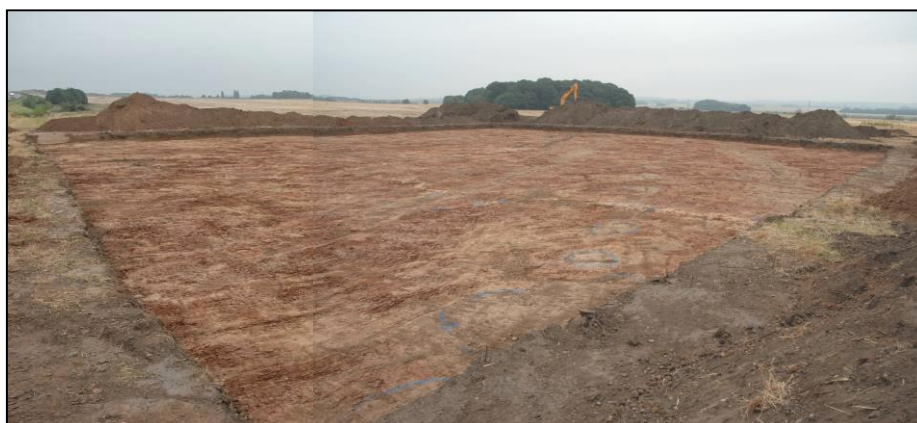
Plate 2: Composite view of the main north-western excavation area in Area 1 at the conclusion of machine top- and subsoil stripping, looking east and south-east.
