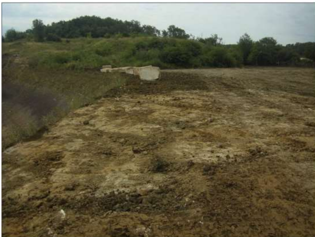
Looking south along the east boundary of Phase III
