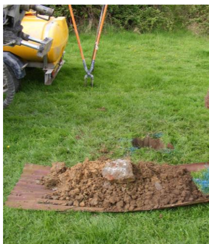
PI. 1: Borehole, looking N
