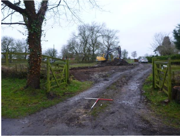
Pl. 1: General view of stripped Car Park Area, looking NNW
