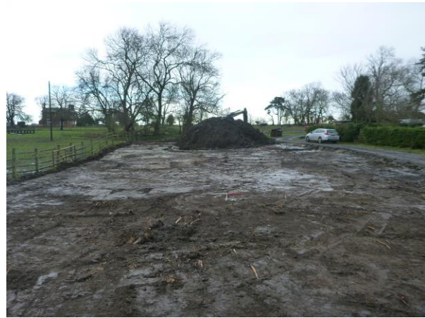
Pl. 2: General view of stripped Car Park Area, looking N
