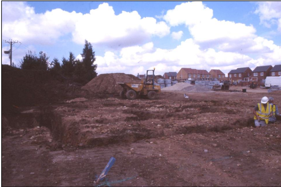
Plate 1: General view of site looking south west
