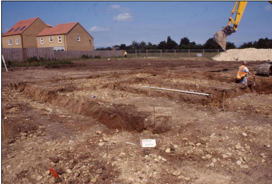
Plate 2: General view of site and house plot 51 looking north east
