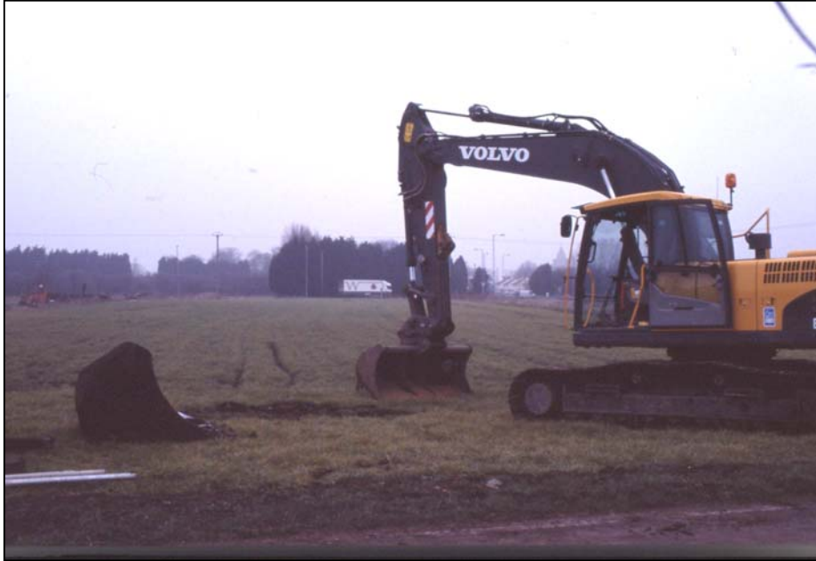
Plate 1: General view of the site looking north
