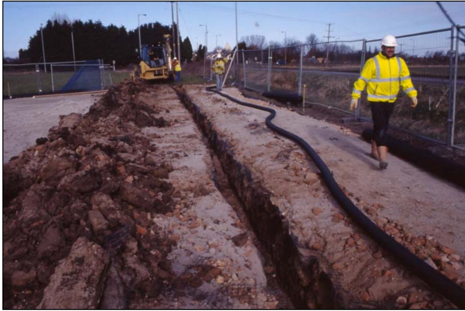
Plate 3: General view of cable trench looking north
