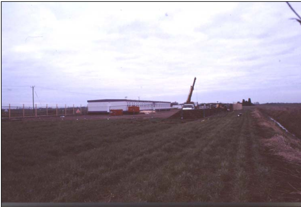
Plate 6: General view of compound showing offices looking south
