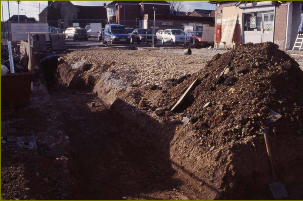
Plate 5: Foundation trenches at front of the development, looking west.
