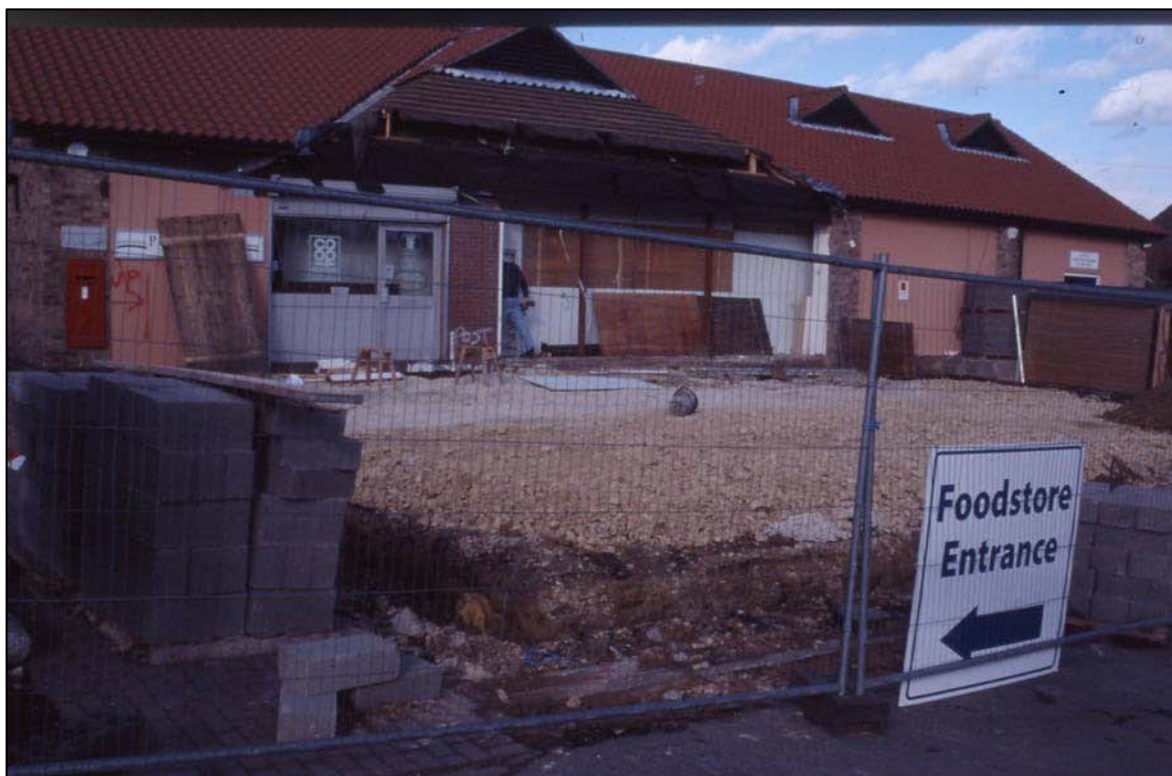
Plate 1: View of Co-Op store, looking north-north-east.
