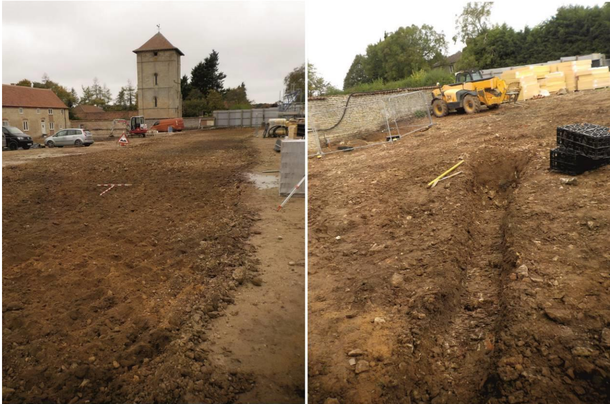
Plate 1: Working shot looking west, showing finished excavation monitored on 13/10/2020.
