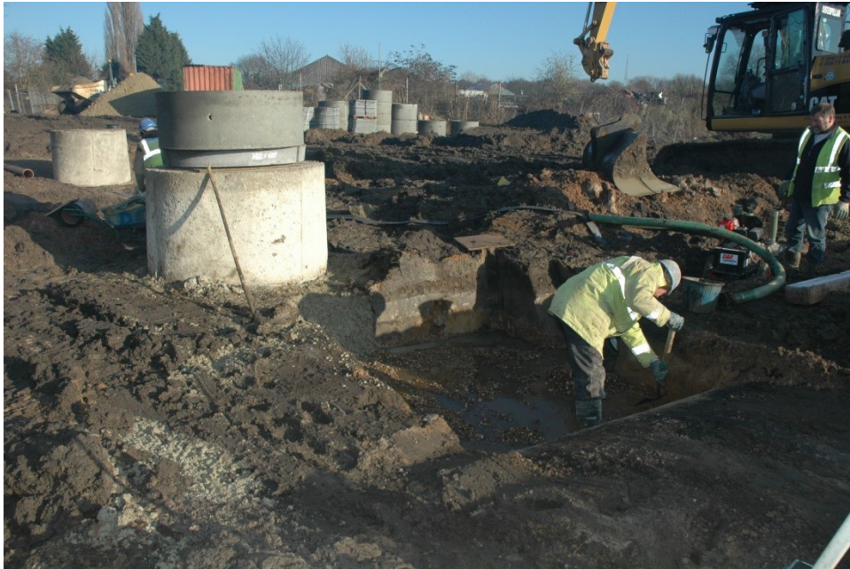
Figure 45: Drain Trench photographed on 18th January
