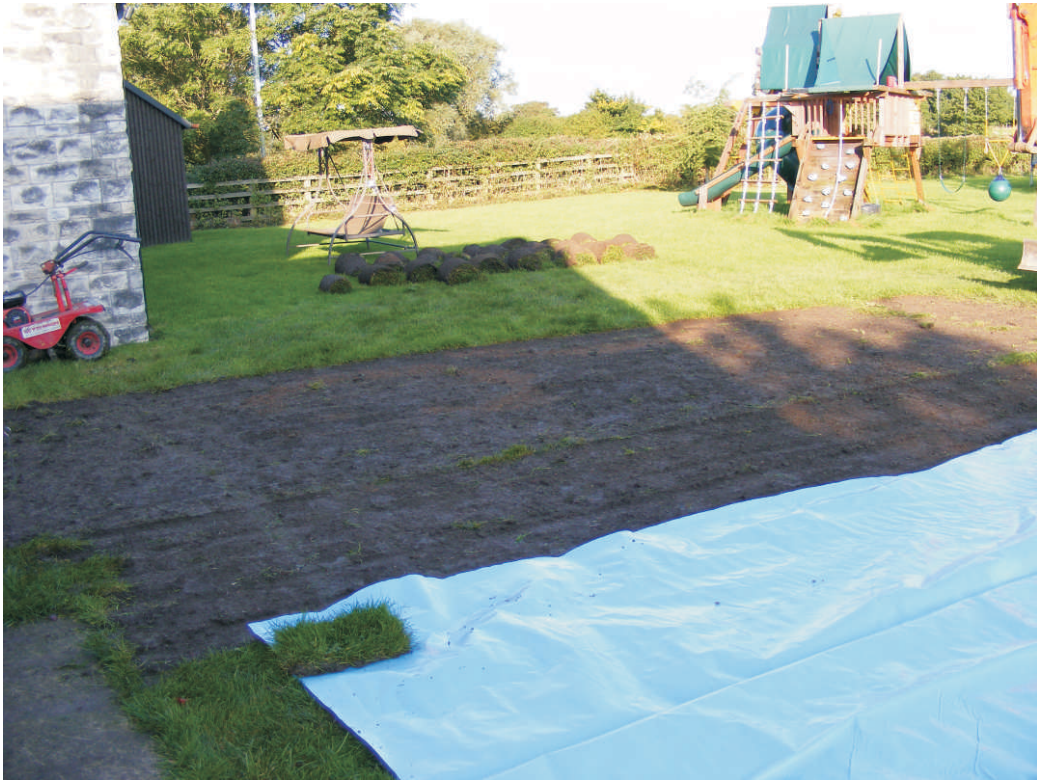
Photo No.1 Location of evaluation trench prior to excavation, looking towards the northwest.
