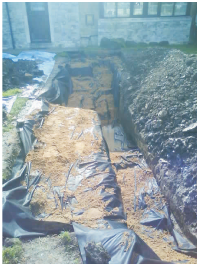
Photo No.6 Evaluation trench being re-instated, archaeology covered with terram , looking south. Photograph by Mr R. Whittaker
