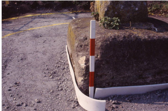
Plate 1: The cross shown surrounded by concrete. The damage to the base can be seen on the front right corner.
