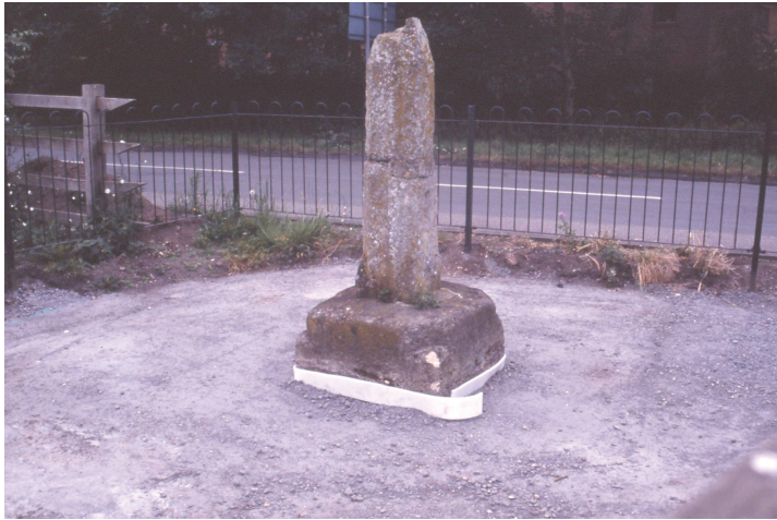
Plate 1: The cross shown surrounded by concrete. The damage to the base can be seen on the front right corner.
