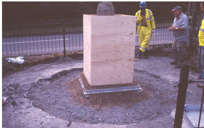
Plate 3: Remedial works being carried out by hand once the wooden shuttering had been erected.
