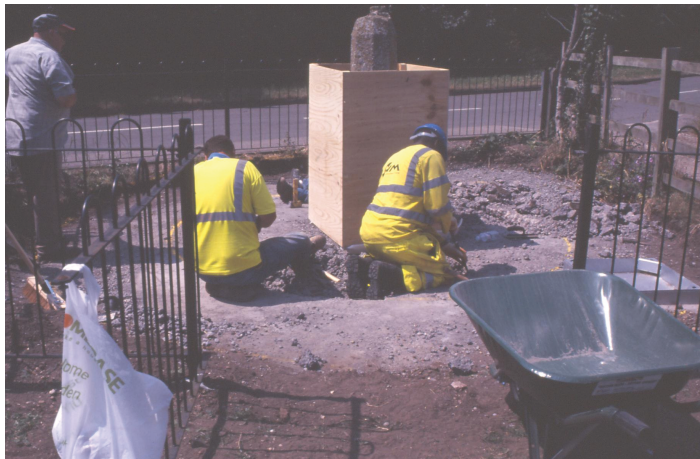
Plate 3: Remedial works being carried out by hand once the wooden shuttering had been erected.
