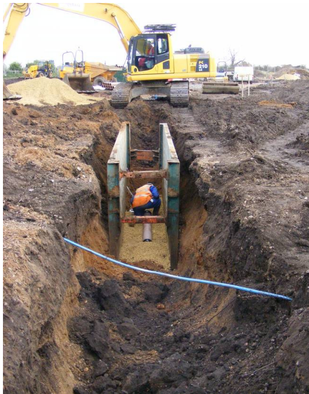
Plate 12: Trench 2 during excavation by the contractors (looking north-west).
