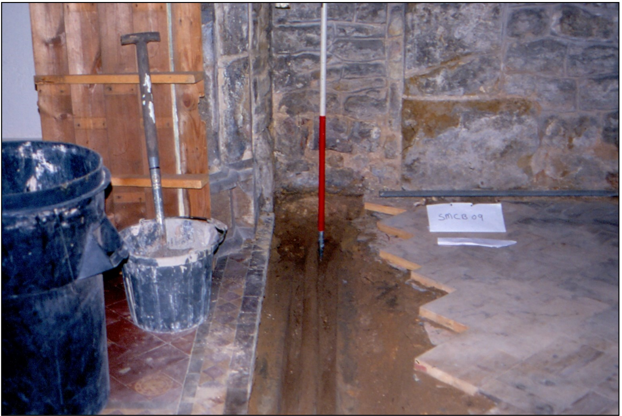
Pl. 3 The pipe duct extended to the west wall of the nave. To the north (right), the abrupt change in the stonework is at the south-east corner of the earlier east wall of the tower (looking west, scale 2m).
