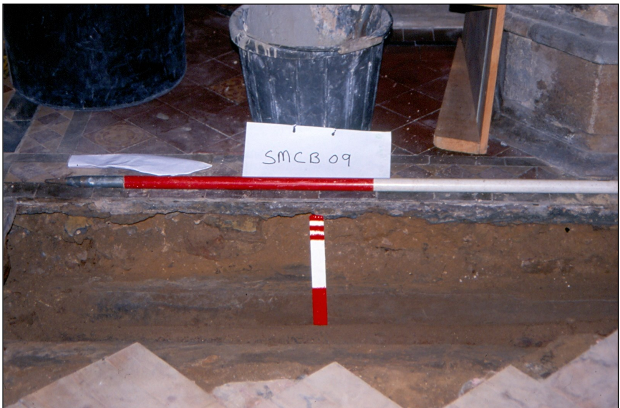
Pl. 2 South face of the re-excavated duct, with the low walls of the concrete lined duct visible at the base of the excavation. The 19 th century floor tiles have been laid above a layer of demolition material (101), which may extend behind the duct. (Looking south, scales 2m and 0.25m).
