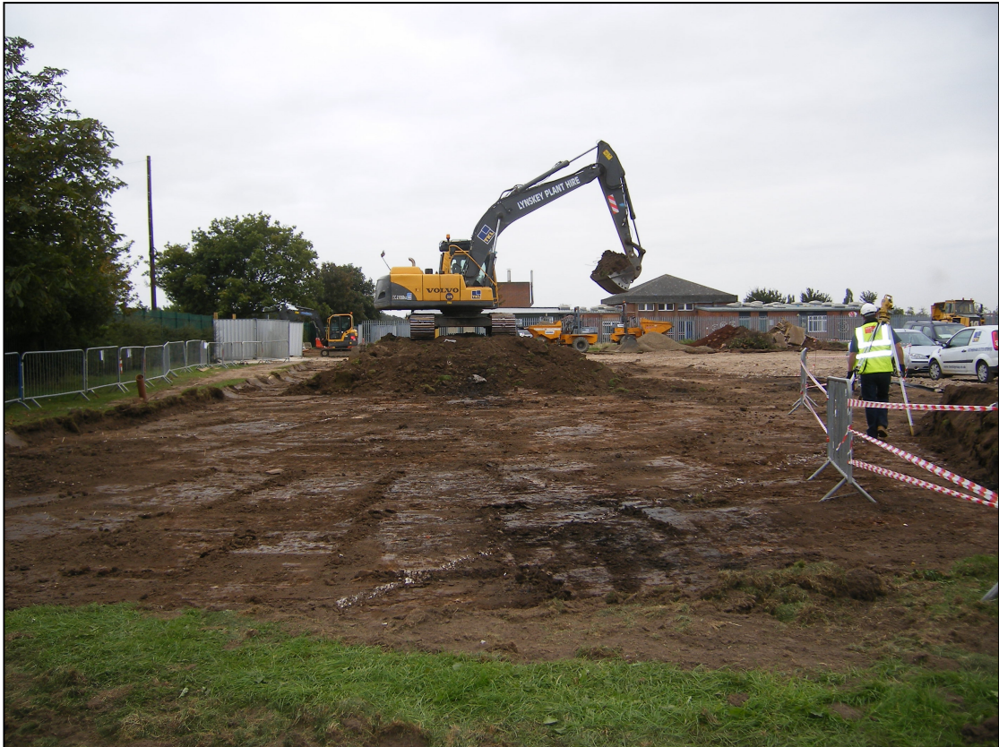
Pl. 10 The contractors' site compound was stripped with an untoothed bucket, but even in these conditions no archaeological features were identified (looking south; the pipe trench beside the eastern boundary can be seen).
