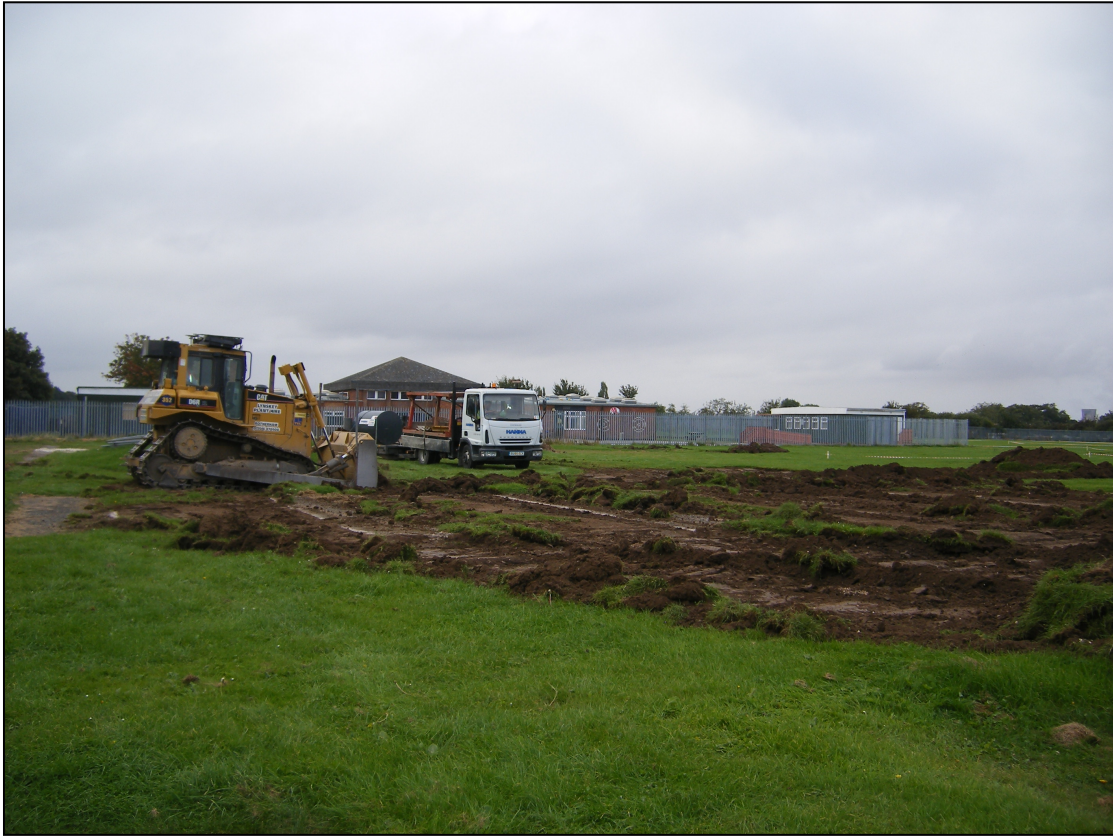
Pl. 3 Much of the development area was stripped of topsoil with a bulldozer (looking south-west).
