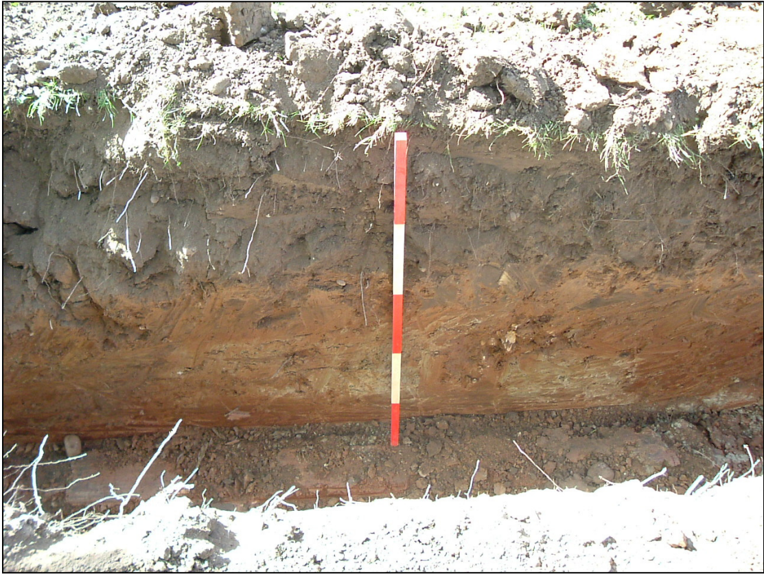
Pl. 9 Topsoil and natural clay deposits visible in the sewer trench face (scale 1m).
