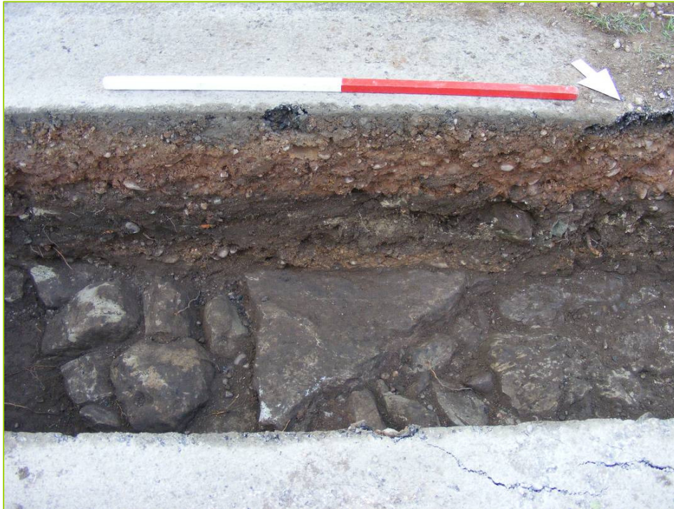
PI. 9 Stone wall/rubble (303) near the churchyard entrance, seen within the pipe trench. Looking south, scale 1m.
