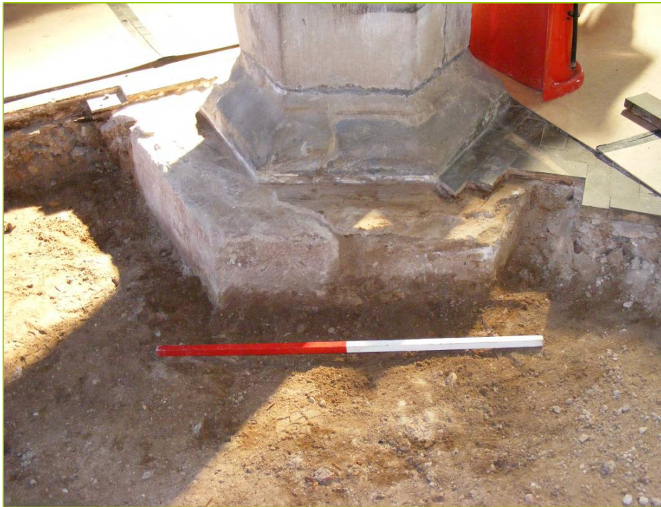
PI. 4 Mortared sandstone base (116) of the south-west arch pillar (looking south, scale 1m).
