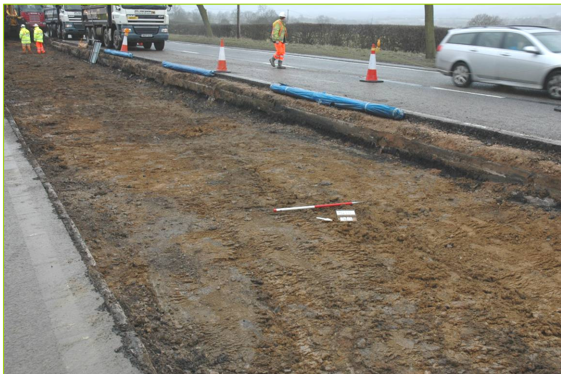
Plate 4: Crossover Area 5 showing stripping completed. The natural substrate can clearly be seen.
