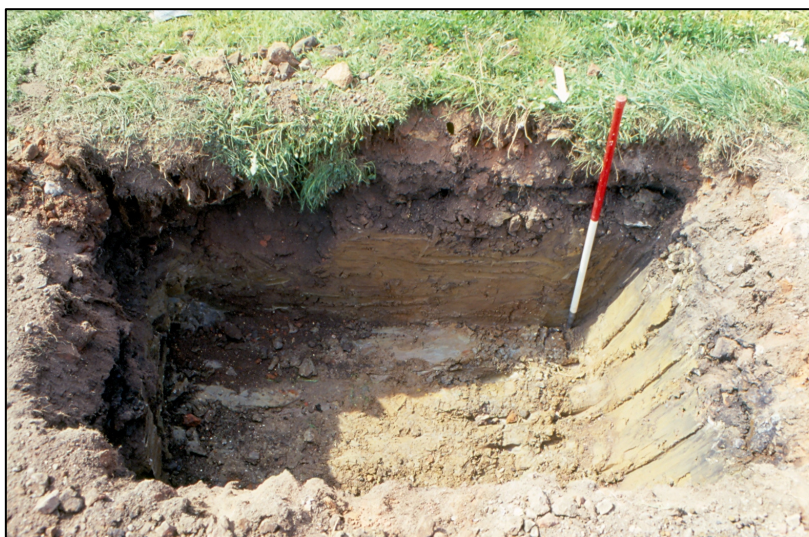
Pl. 12 To the south of the house, a percolation test pit encountered thick imported rubble directly above weathered boulder-clay natural. Scale 1m).
