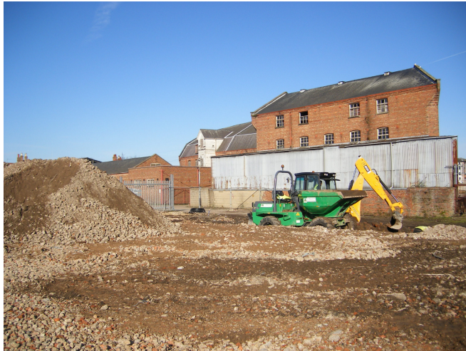
Plate 1: General View of site Looking north-west.
