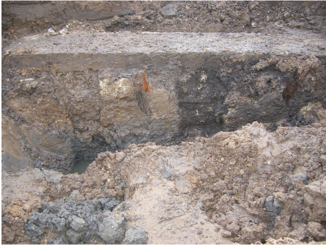
Plate 5: Concrete structure (115) looking south-west.
