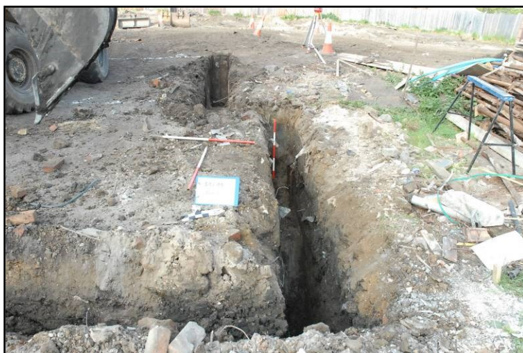
Plate 3: Plot 2. Foundation trench (Frame 14) looking south.
