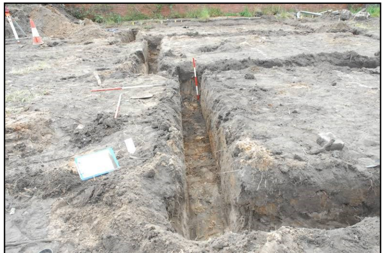
Plate 5: Plot 4. Foundation trench (Frame 9) looking south.
