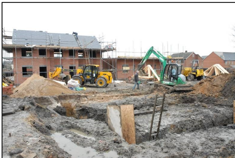
Plate 1: General view of site looking west, incorporating Plots 3 to 7.
