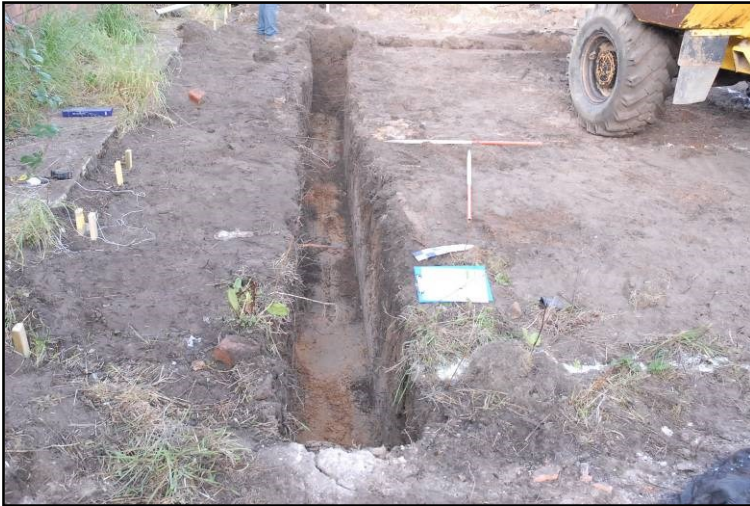
Plate 4: Plot 3. Foundation trench (Frame 2) looking west.
