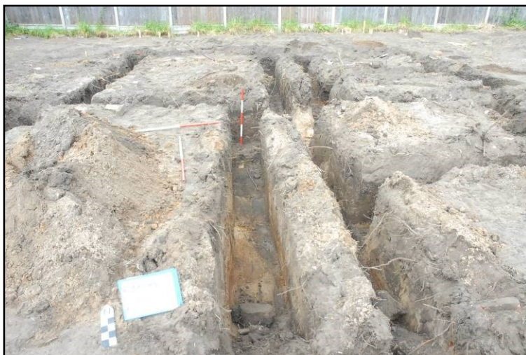
Plate 6: Plot 6. Foundation trench (Frame 13) looking north.
