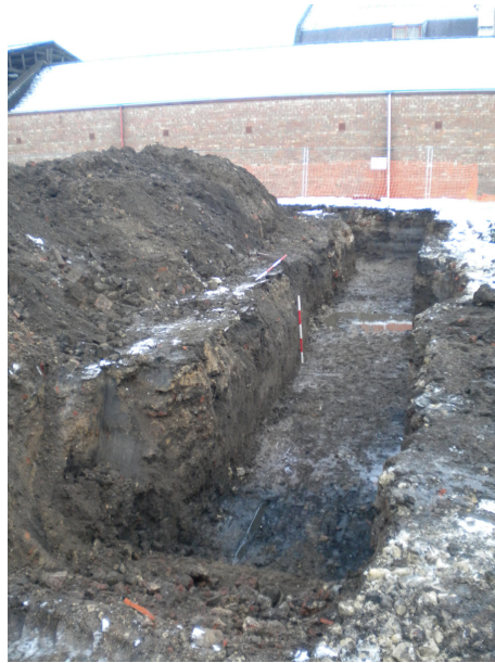
Plate 2 Post excavation Trench 2 looking northeast
