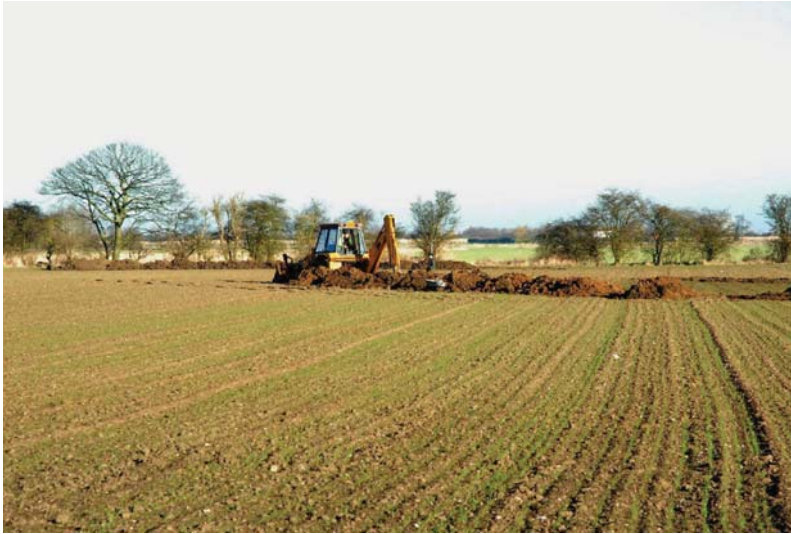
Plate 1 General shot of the site looking towards Trenches 1 and 2, looking north-northeast
