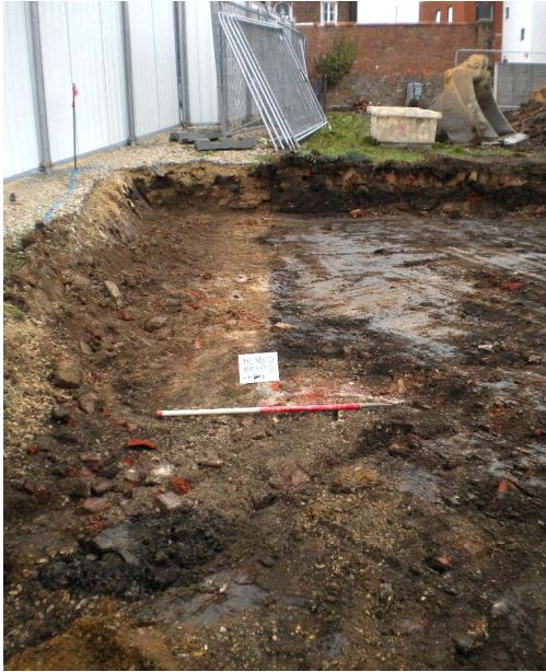
Plate 5 Wall (102) looking west
