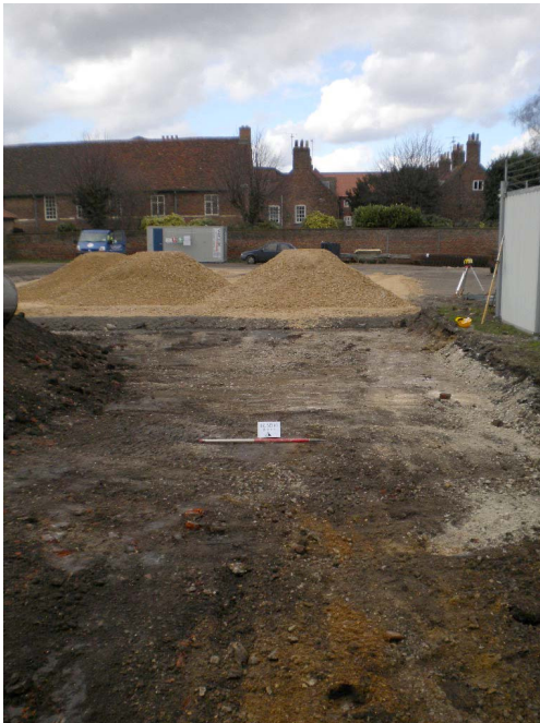
Plate 3 Northern end of site after excavation
