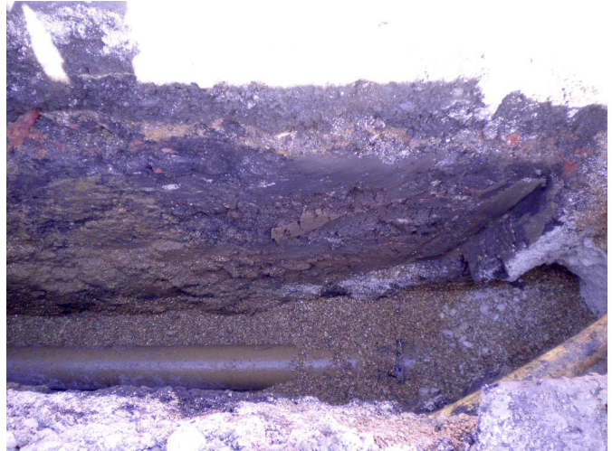
Plate 6 Layers (109) and (110) in drainage trench looking north
