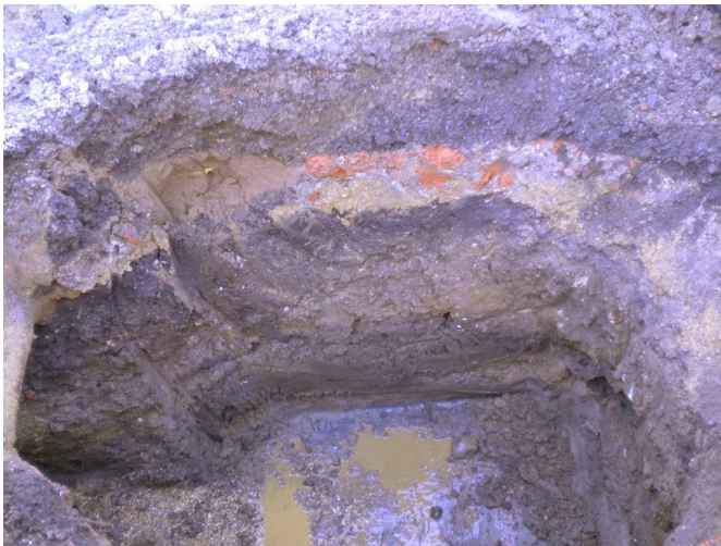
Plate 7 North facing section in drainage manhole (fig. 7)
