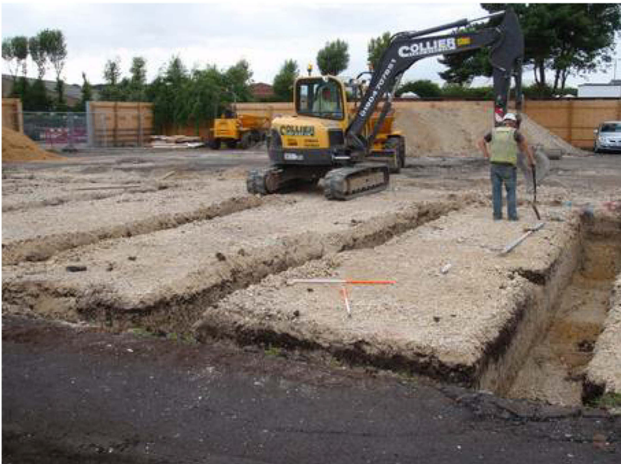
Plate 4 Plot 2 after excavation looking northwest
