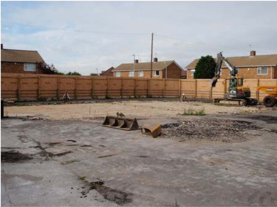
Plate 1 General view prior to construction works, looking southwest
