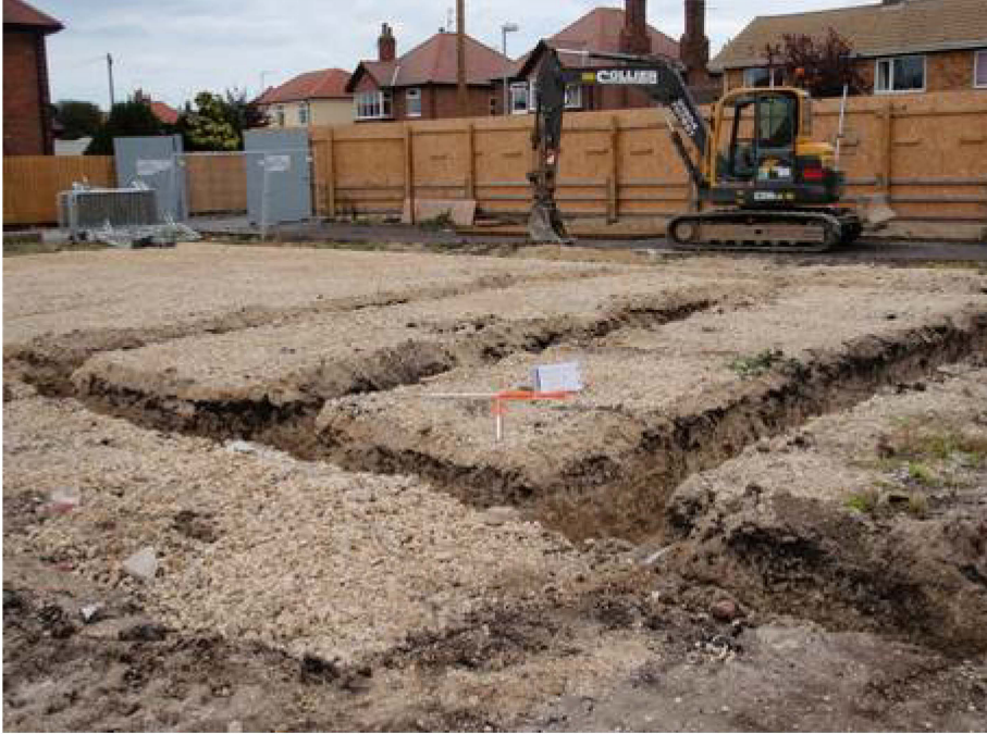
Plate 3 Plot 3 after excavation looking southeast
