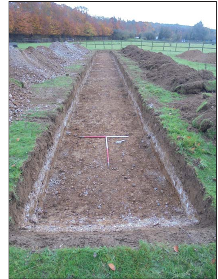
Trench 3, looking south-east (scales 1m)
