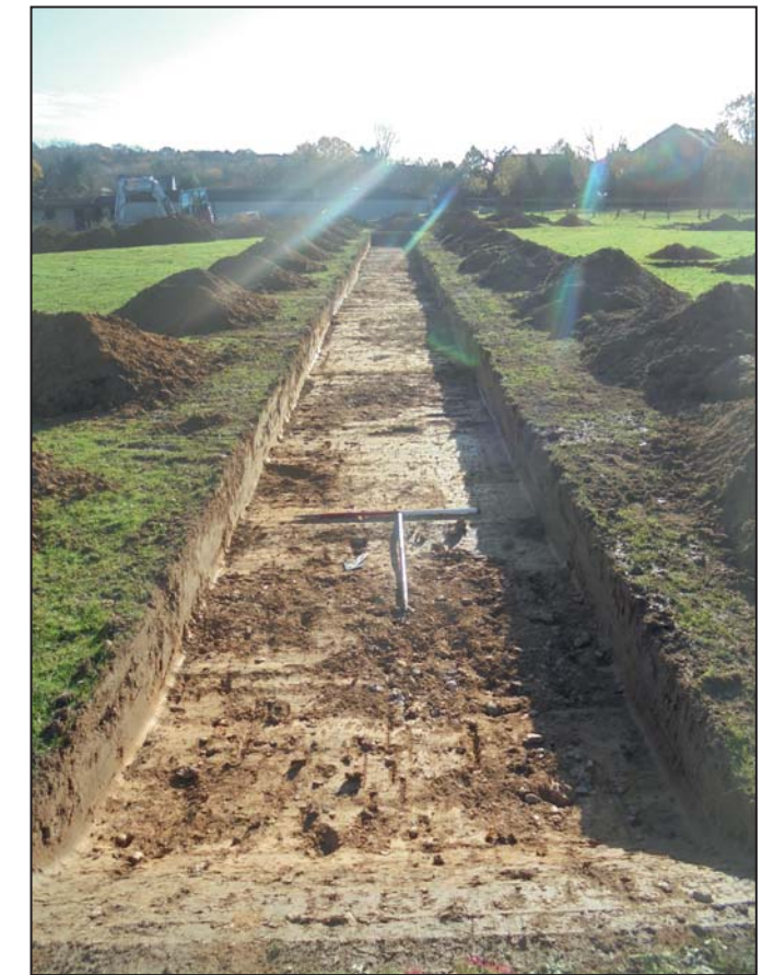
Trench 29, looking south-east (scales 1m)
