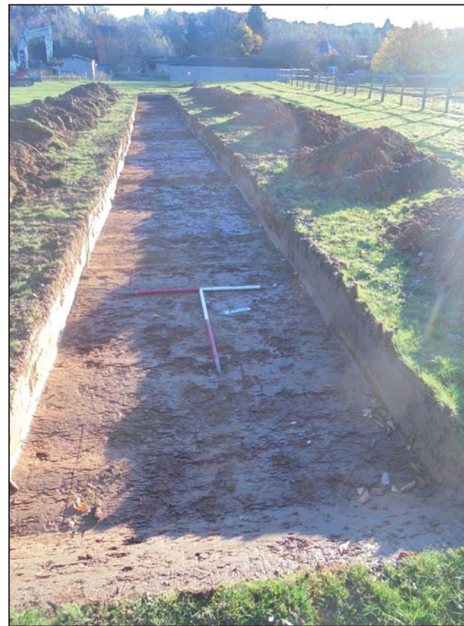
Trench 31, looking south-east (scales 1m)
