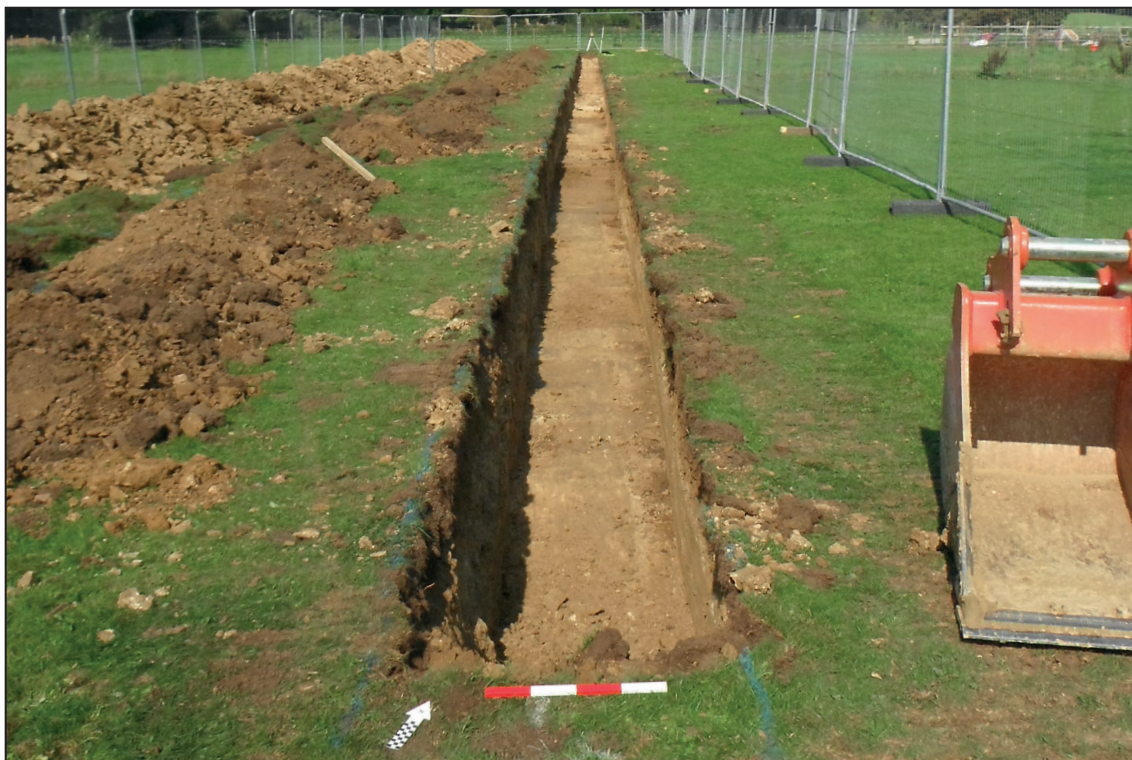
Area 2, looking north-west (0.4m scale)
