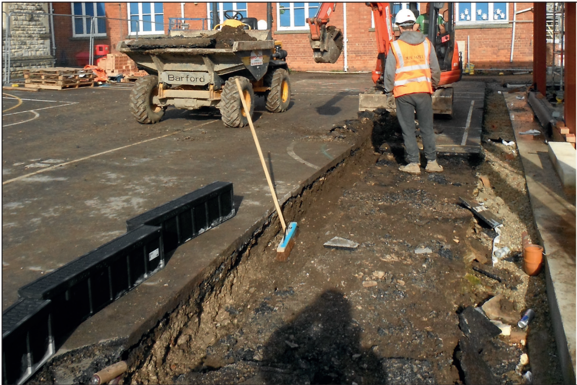
Trench 18, looking north-west
