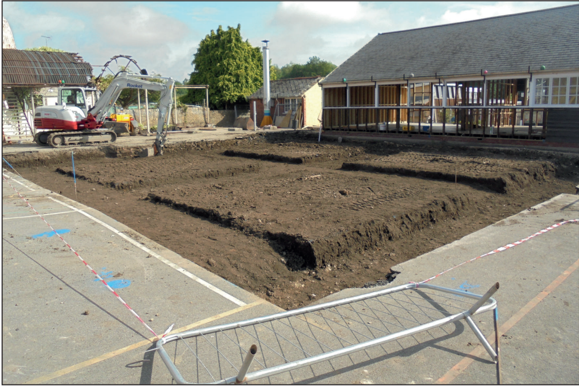
Trench 7, looking north-east
