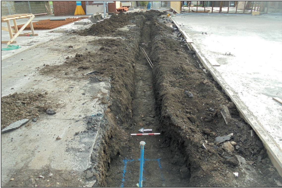
Trench 8, looking east (0.5m scale)
