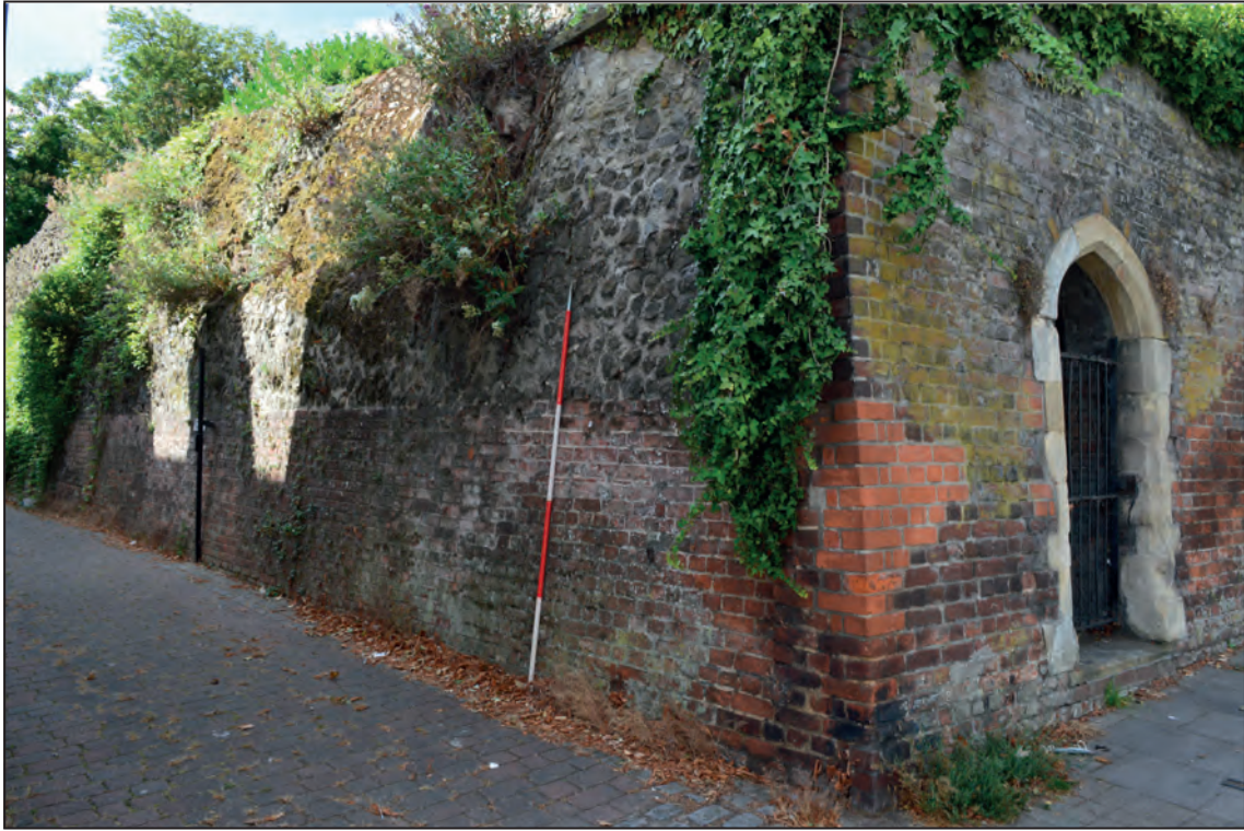
Underpinning of wall opposite East Hill excavations, looking south-west (2m scale)
